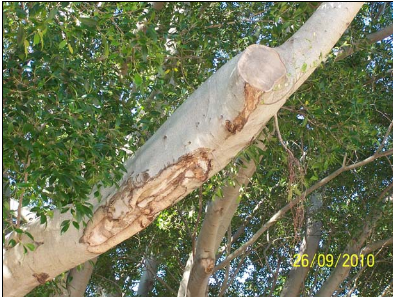
Figure 10 High vehicle impact creates a hazard for the tree 12012. This branch arises from a codominant union at the base of the tree and hitting this branch could result in whole tree failure.
